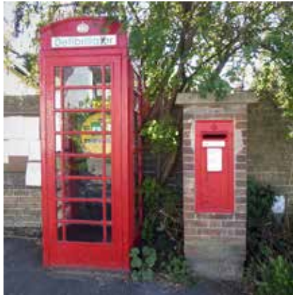
Figure 35: Grade II listed K6 Telephone Kiosk
