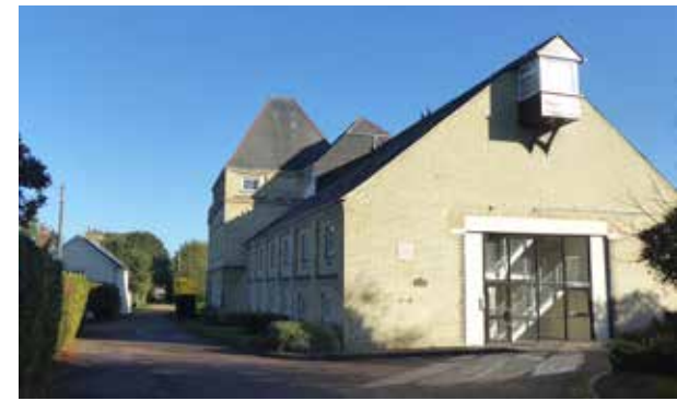
Figure 54: Former Fordham Maltings, Green Lane/Station Road
