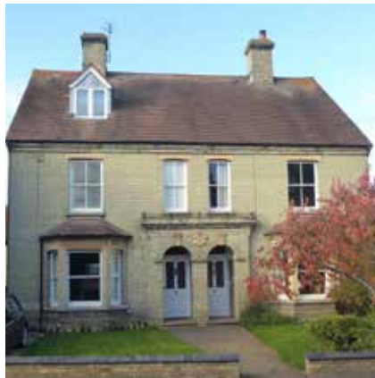
Figure 28: 86 and 88 High Street
