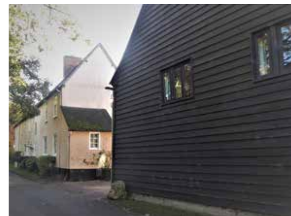
Figure 46: Example of weatherboarding, Ringstead Farm
